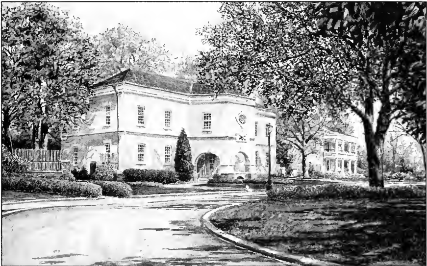
Historic Payne Hall (left) and Rains Hall
